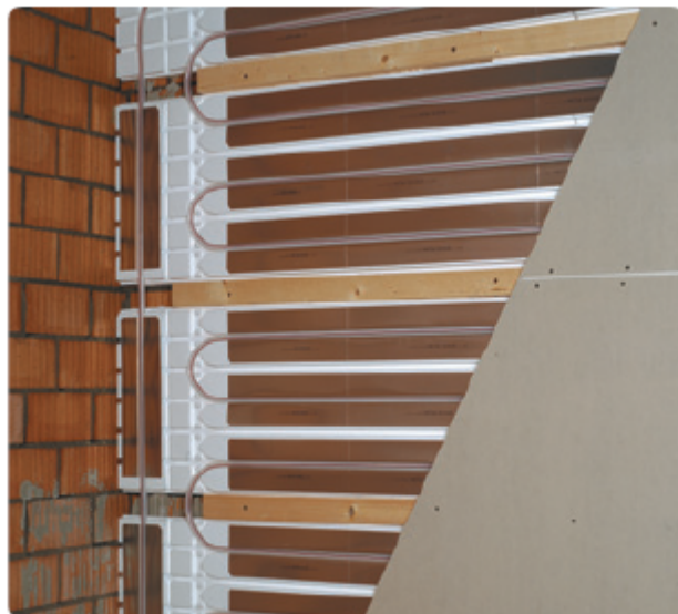
Uponor Siccus wall heating installation with drywall panels
