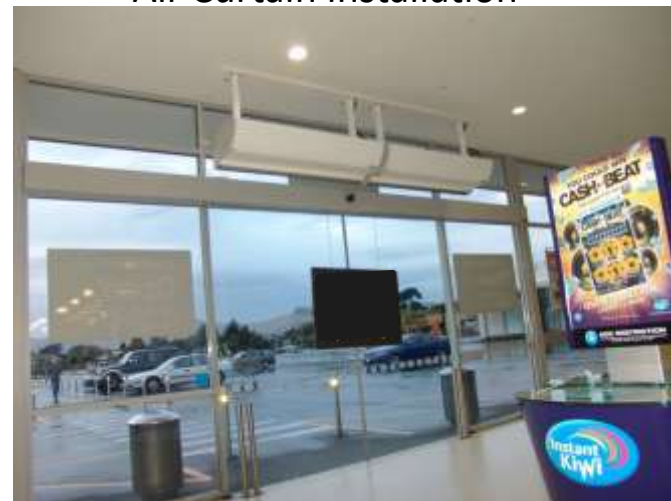
Air Curtain installation
